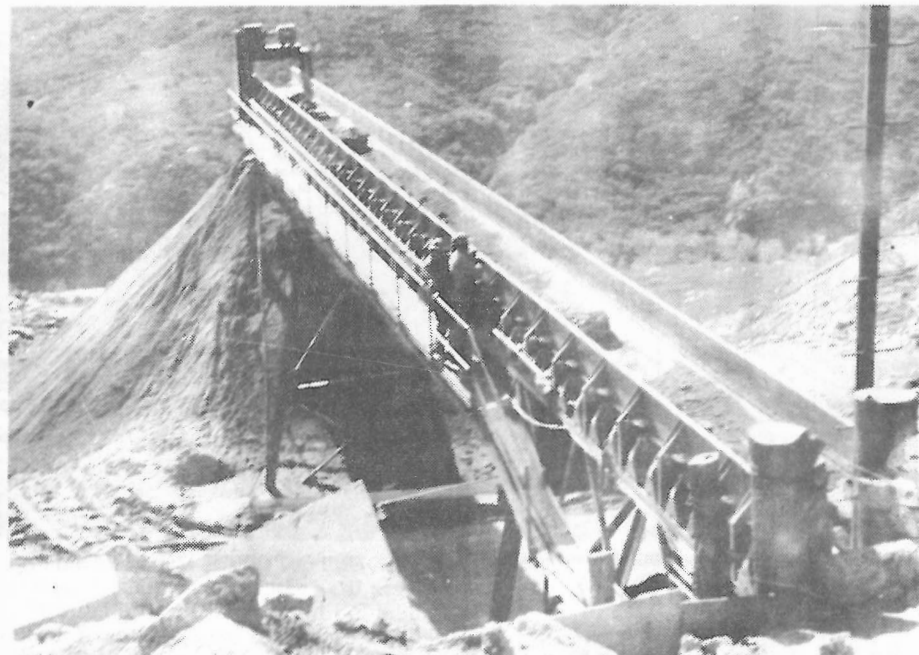
Huge conveyor belt that is slowly moving mountain from one side of Hwy 80 to other.
